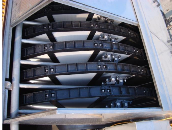
Picture 2: Installed filter elements by GKD.
