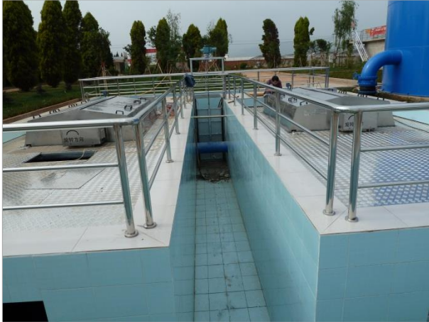
Picture 1: Filter in a sewage plant.
